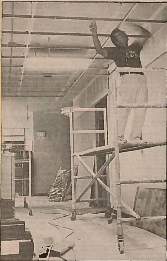
Worker Frank Evans of Tahoe City, Calif., tapes off newly installed ceiling supports. Remodeling has included putting a lower ceiling into the building. Work is expected to be finished in about two weeks.
